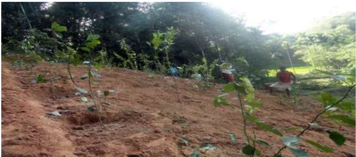
Image-8: Hill slope plantation for erosion protection
